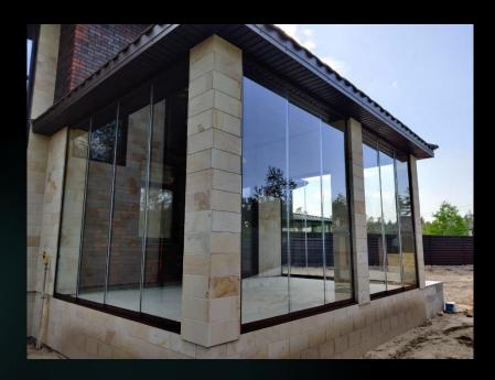
Material: Aluminum - glass Glass type: 8/10 mm tempered Profile color: Anodized - RAL
